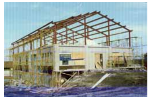
Photo (above): Construction of “Ontario Place Hotel”. Photo taken March 1990.
